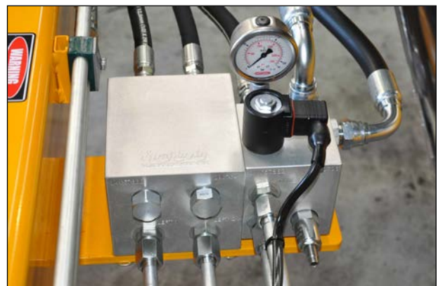
Hydraulic Control Block
